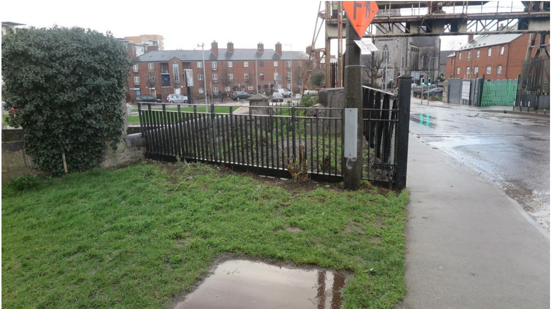
After East facing south side Samuel Beckett Bridge
