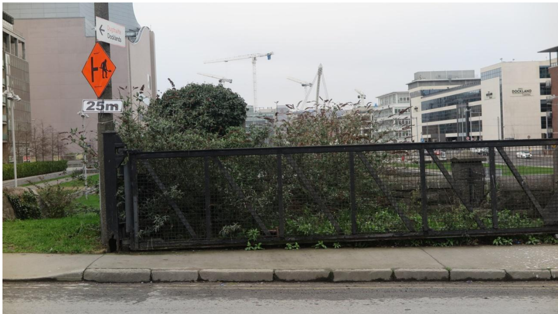
Before South facing Samuel Beckett Bridge
